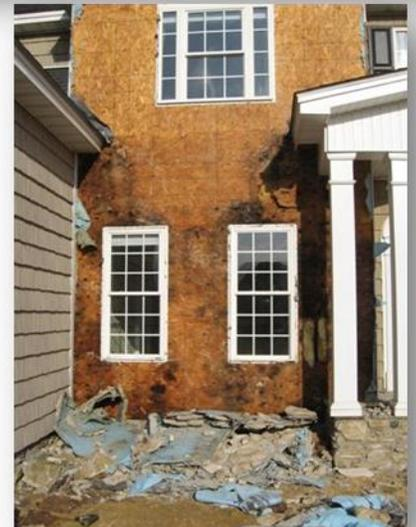
applied directly to framing in order to prevent moisture decay. Like the EIFS system, I expected that a drainage barrier was going to be needed behind the stone. For direction and guidance, the Masonry Advisory Council was contacted and asked if they had either specifications or standard details on adhered stone masonry. They did not but referred me to the Brick Institute of America's detail for adhered brick veneer (shown at bottom right of page 2).
